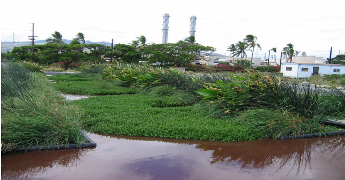
Constructed wetland for removal of pollutants
